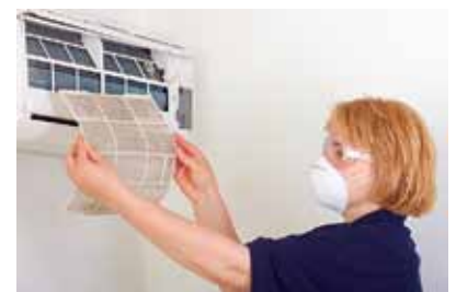
Arrange regular cleaning of your air conditioning unit to maintain efficiency and capacity.
